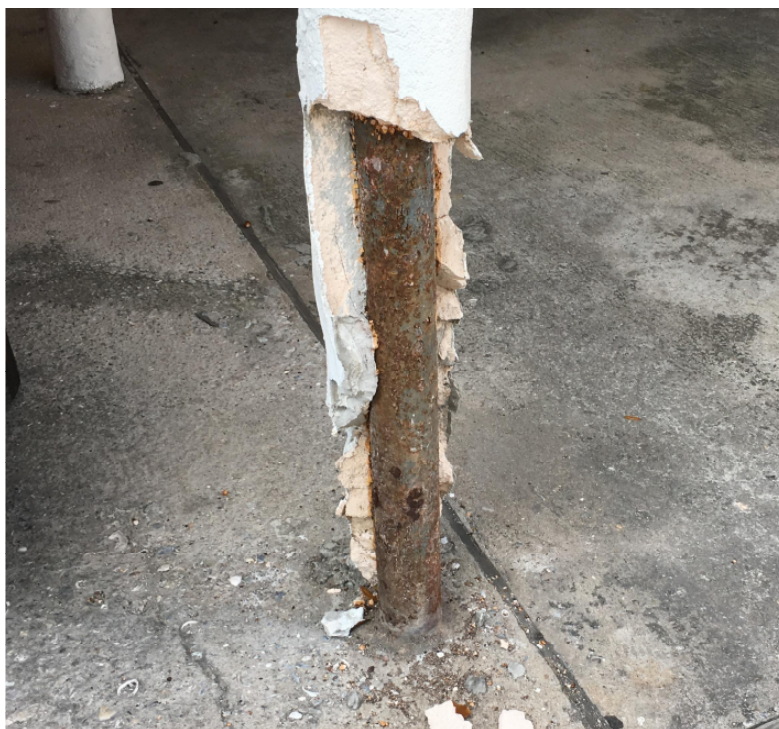
Photo 9 – Corrosion of Column at Building 3
