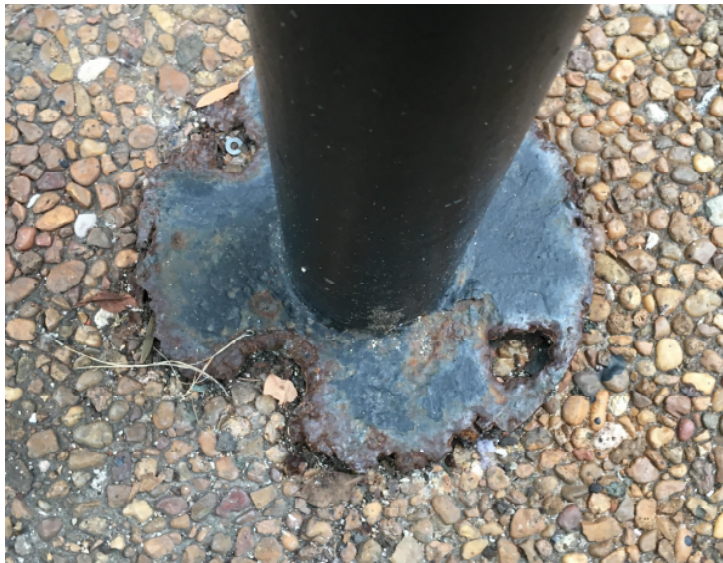
Photo 14 – Corrosion of Rear Stair Baseplate
