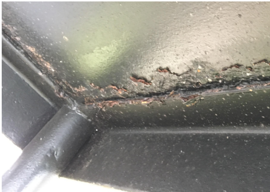
Photo 13 – Corrosion on the Underside of Rear Mid Landing
