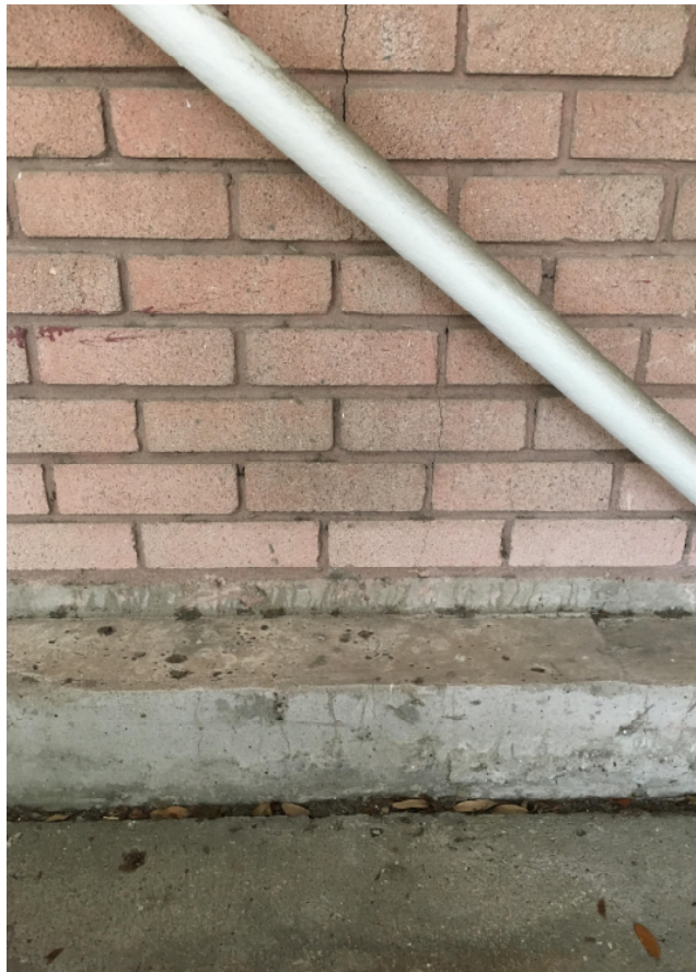
Photo 11 – Crack in Masonry Wall at Building 3
