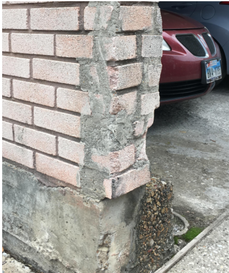
Photo 10 – Spalling of Brick on Southeast corner of Building 3
