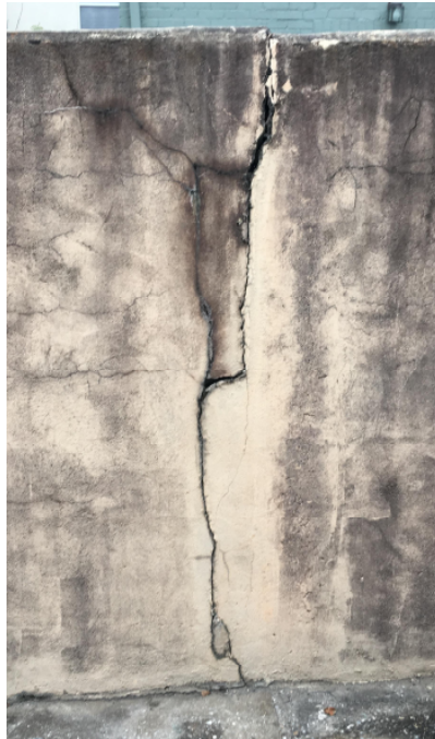
Photo 16 – Major Crack in West Perimeter Wall
