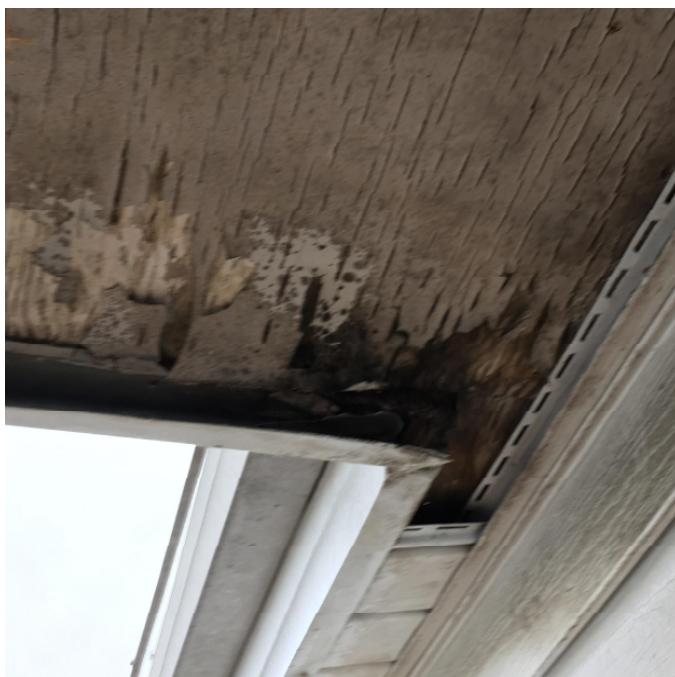
Photo 5 – Condition of Soffit on Underside of Roof Overhang
