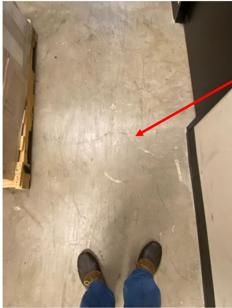
Crack in slab outside of printshop
